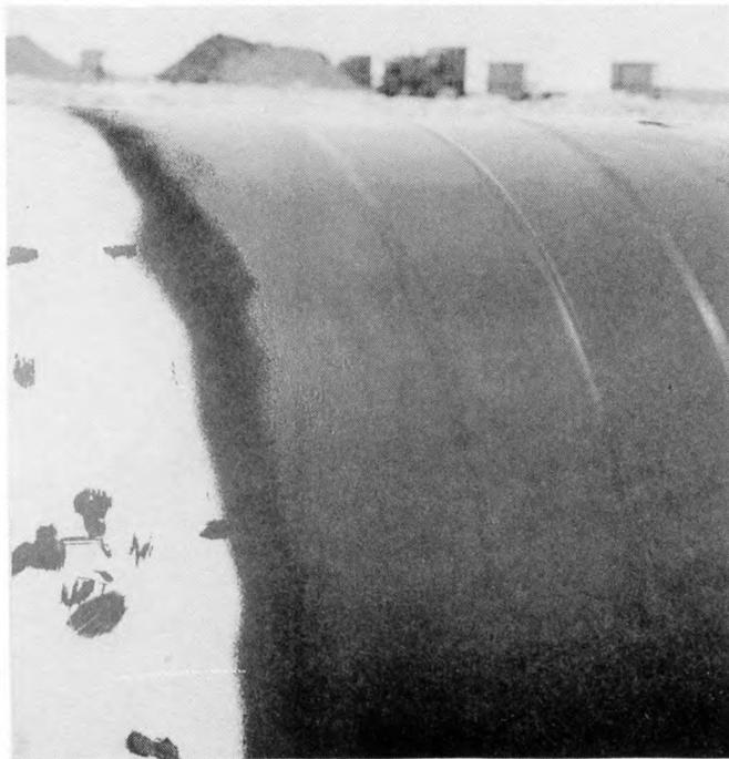
**Figure 6, Coated field weld Joint**
